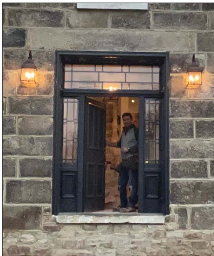
The relocation and reconstruction of the Hogg Stone House from Tremaine Road onto King Street Milton is nearly complete. Occupancy is expected by the end of February. Here, Manuel is installing the front door and transom, which was restored and re-installed in the new house.
