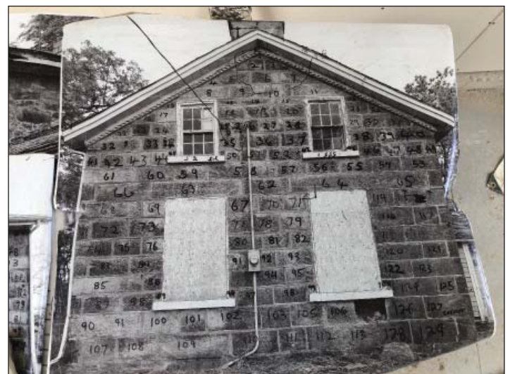
Above and below: The stonemasons are reconstruction the house brick by brick. Extensive photographs on the house were done on Tremaine Road and each brick was carefully numbered on the photographs and on the bricks themselves.
