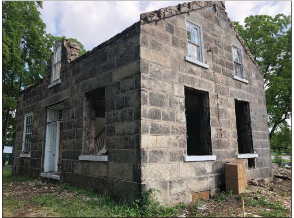
The careful dismantling of the Hogg stone house on Tremaine Road has begun. It will be rebuilt on King Street in Milton. The process will take about a year.
