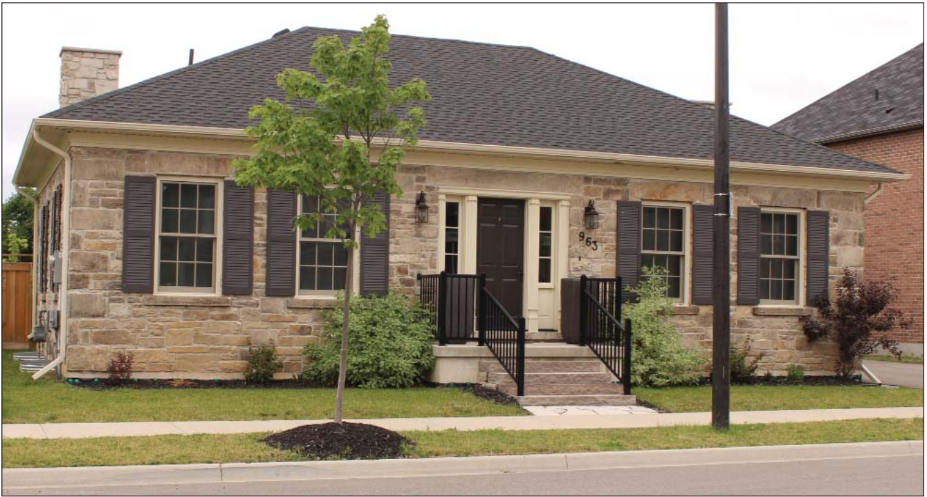
Featherstone House was sympathetically de-constructed and re-built as a frame house with a stone veneer at the edge of Featherstone Park in Milton.
